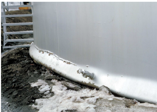
Figure B.5-4 – Elephants’s foot buckling. Anchorage earthquake in 1964, M 9.2.
