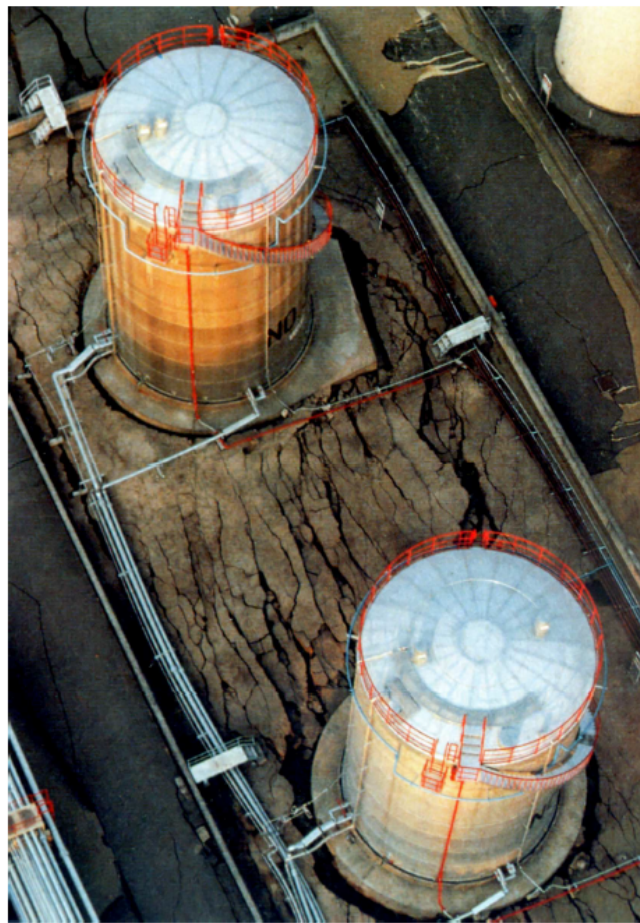
Figure B.5-1 – Soil liquefaction around tanks. Kobe 1995 earthquake, M 6.7.
