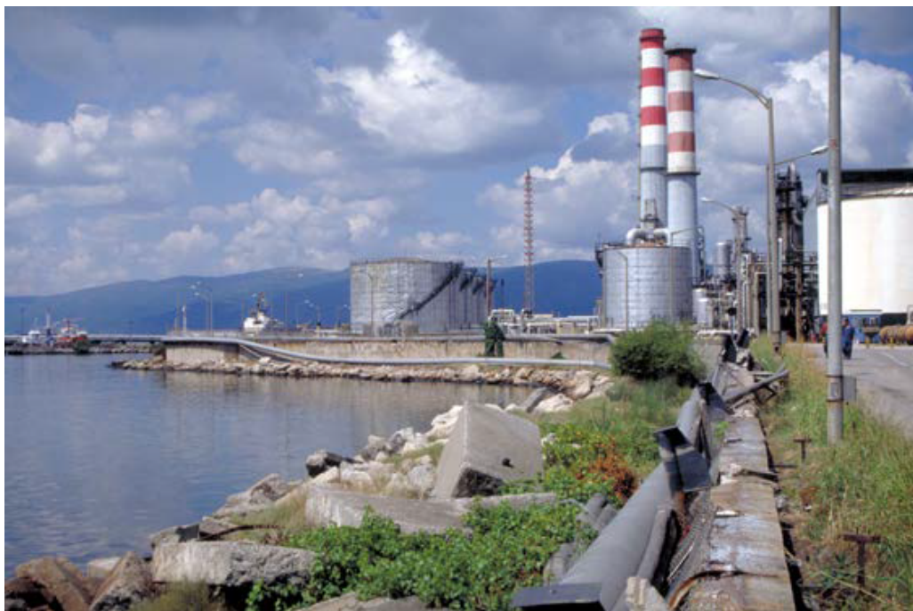
Figure B.6-2 – Displacement of a piping system. Izmit (Turkey) 1999, M 7.4.
