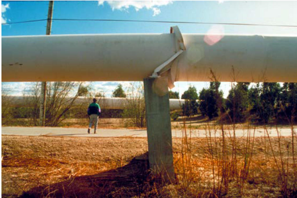
Figure B.6-3 – Movement of supports due to soil liquefaction. Northridge 1994, M 6.7.
