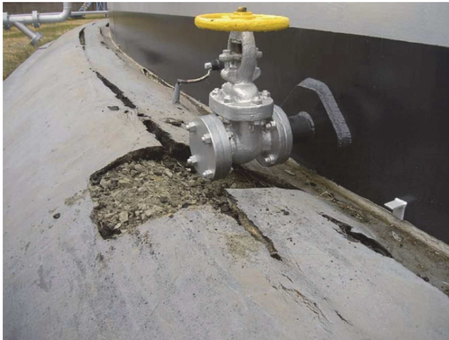
Figure B.5-2 – Tank settlement due to liquefaction around the tank foundation.
