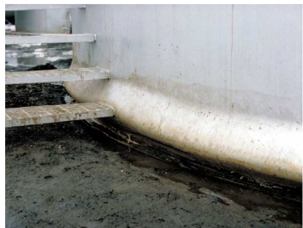
Figure B.5-4 – Elephants’s foot buckling. Anchorage earthquake in 1964, M 9.2.
