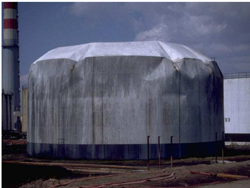
Figure B.5-8 – Sloshing damage to upper shell and roof of a tank. Marmara (Turkey) earthquake 1999, M 7.4.
